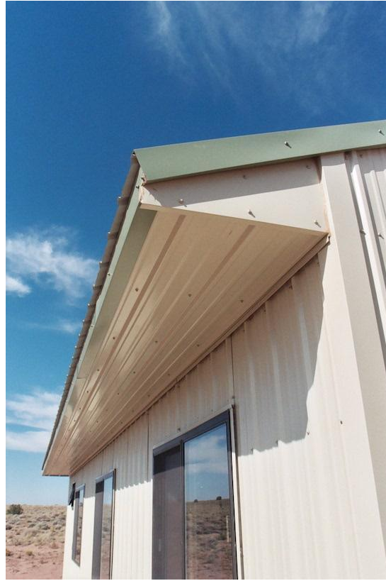
Wrapping all exposed lumber in steel, for zero maintenance
