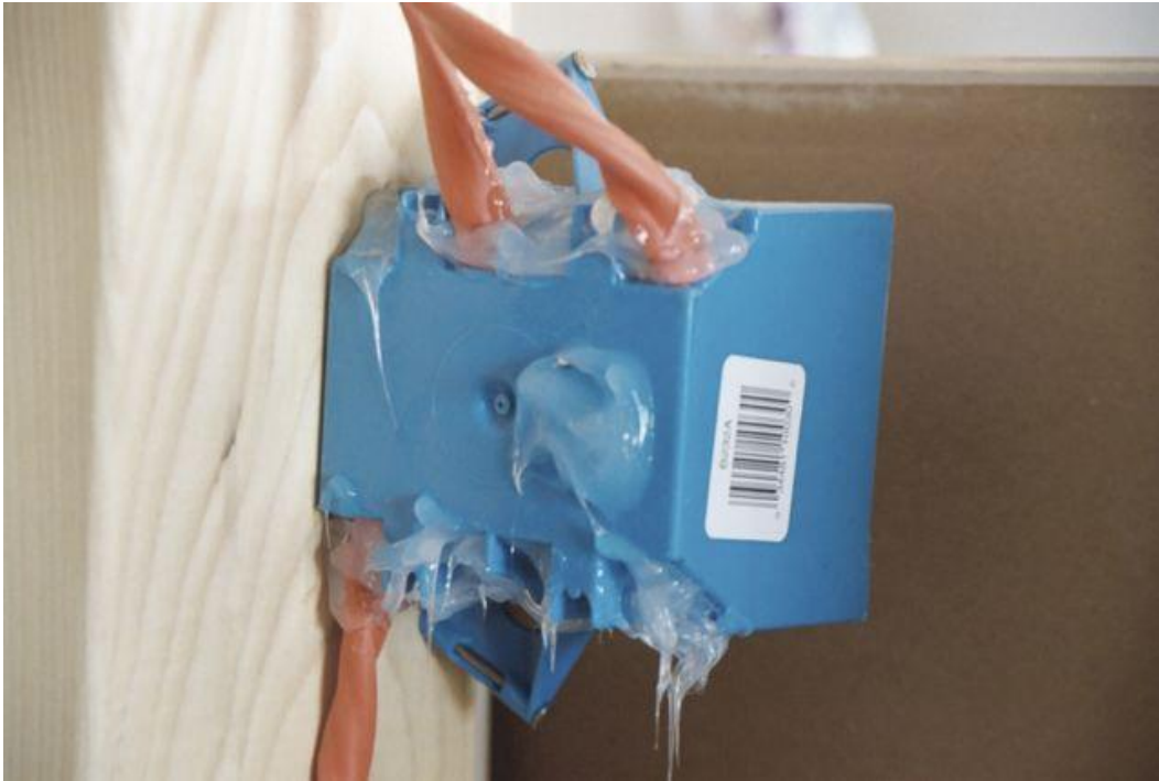
Wall box sealed with silicone caulk. Expanding foam in a spray can works better.
