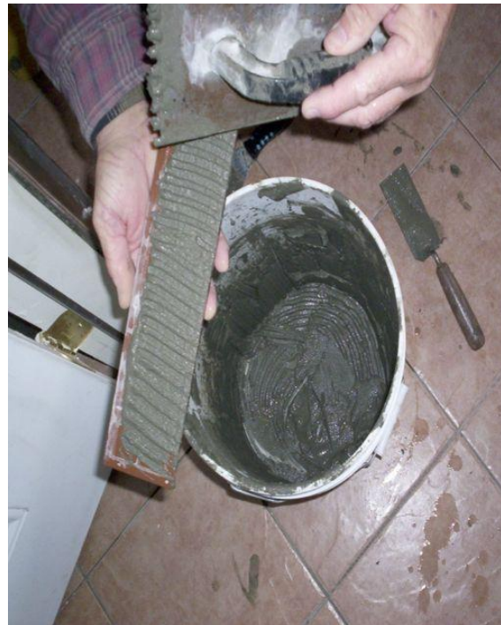
Setting the tile around door and baseboard, using steel mesh (degreased hardware cloth) for extra strength in these areas.
