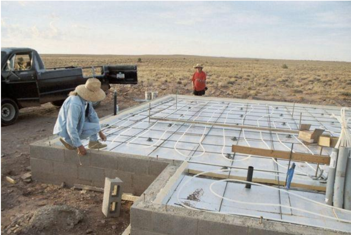
The foundation is ready to be poured. The foam boards, the PEX tubing and the stem walls can be seen.
