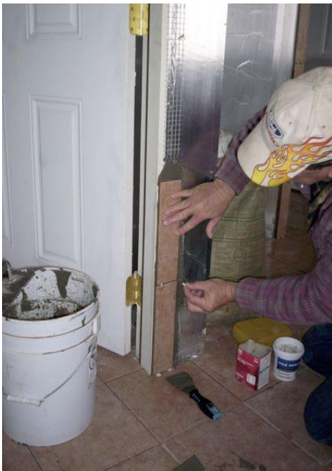
Setting the tile around door and baseboard, using steel mesh (degreased hardware cloth) for extra strength in these areas.
