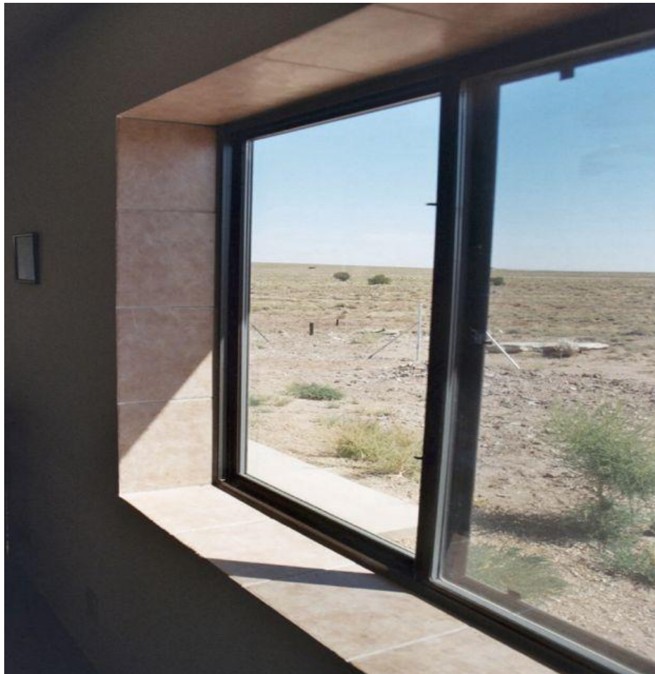
Tile work around the window, with HardiBacker cement board underneath
