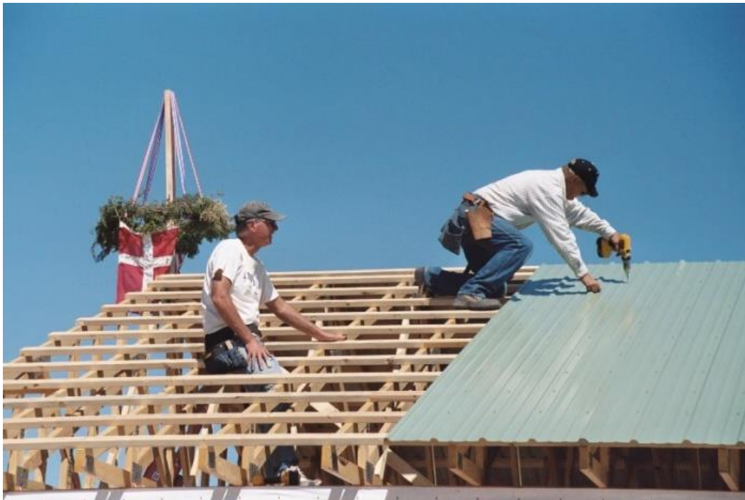
Mounting steel roof panels without decking underneath.
