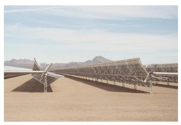
Power plant in Nevada that is similar to the Solana plant. The heat-transfer oil is pumped through the pipes in front of the mirrors.
