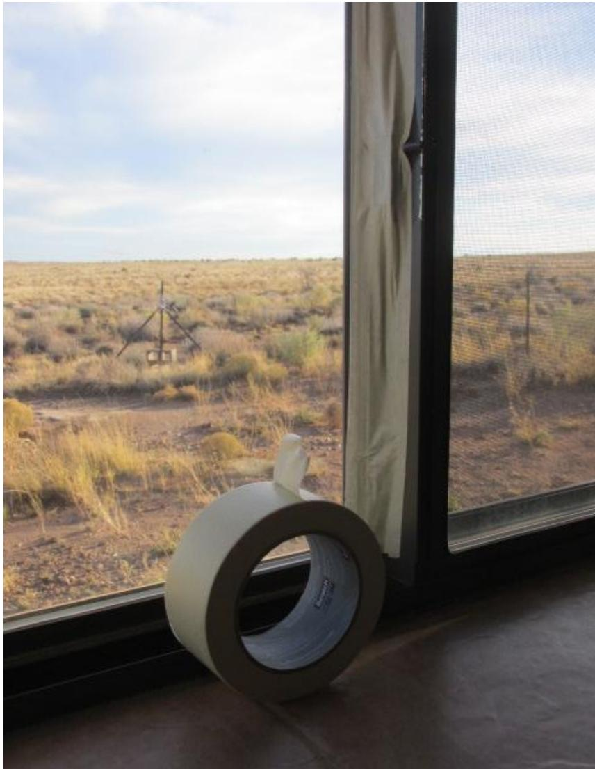
*Masking tape sealing the gap between two window panes that slides horizontally.*
