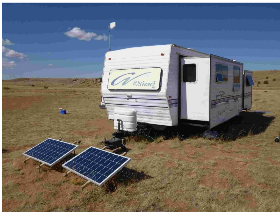
People who can't afford a house sometimes live in travel trailers. A DC-only solar system makes off-grid living more comfortable.
